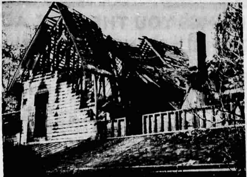
CHARRED REMAINS —After two serious fires, Jacksonville's historic Britt house is left more than a fire-charred skelton. The old home will be destroyed prior to June 1, according to a recent agreement between the Jacksonville city council and Southern Oregon college, owner of the house. Both the council and college agreed the house is a safety hazard and must come down.
