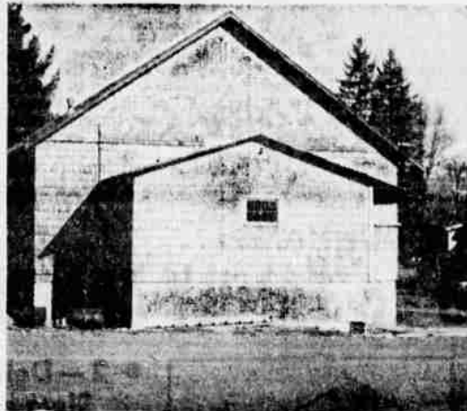
BUTTE FALLS COMMUNITY HALL Work May Be Completed This Year
