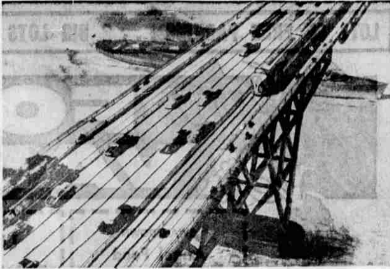
PROPOSED BRIDGE —This is an artist's impression of a section of the proposed 25-mile-long English Channel bridge to link Great Britain and France. The bridge would be 110 feet across, having a five-lane motor highway, two railroad tracks and separate paths for cyclists and motor-
