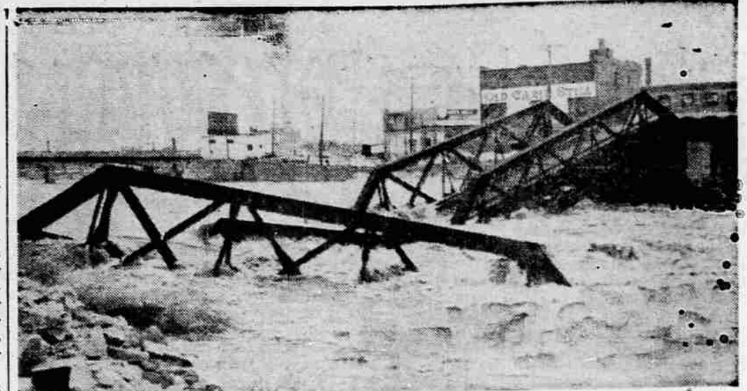
BRIDGE BATTERED —Pressure of ice and S. D., today as the Big Sioux river went on rising water took out a steel span on the a rampage. Rock Island Railroad bridge at Sioux Falls.
