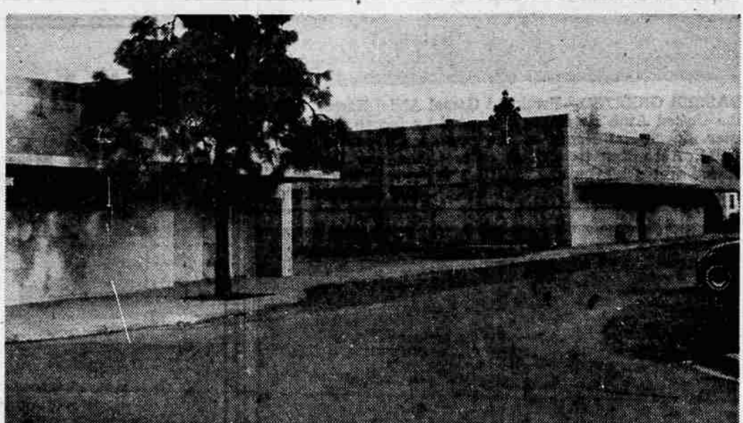
HIGH SCHOOL BUILDING —Above is a renovation in the original high school structure of the space between the music rooms (left behind tree) and the shop rooms (right) where the boys physical education plant will be completed. Completion of the unit will provide seven teacher stations, and another teacher station will be made available by
