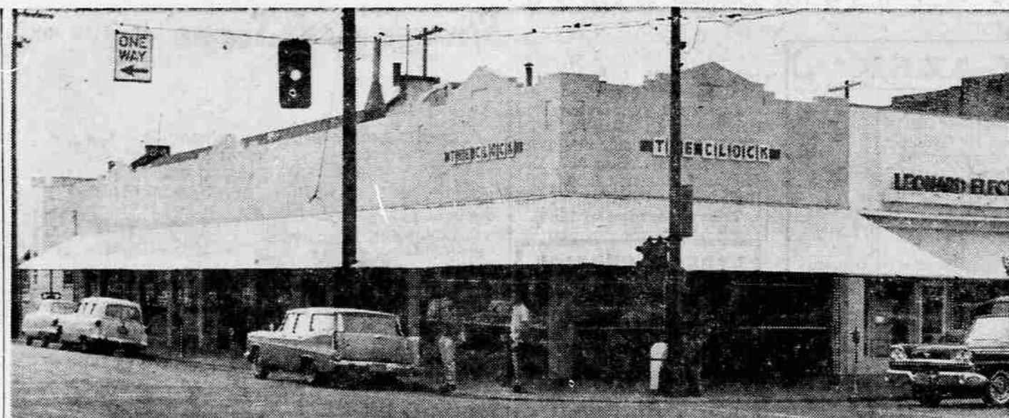
NEW LOOK -The Belle E. Warner building, which includes the Clock restaurant on Main st. and two other recently-remodeled business locations on Bartlett st. in Medford, recently took on a new appearance with the addition of a permanent fiberglass "awning" that extends over the entire sidewalk, offering protection from rain and sun to passerby. Occupying the new business sites will be
