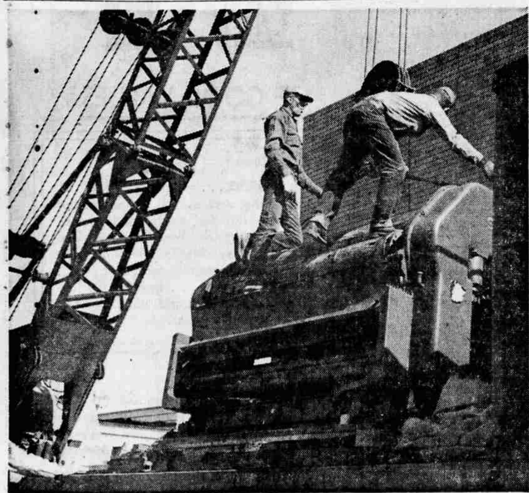
NEW PRESS —One of three sections of the new printing press that will be used to print the Mail Tribune after May 1 was moved into the new press building on Grape st. yesterday, after arriving by freight truck from Plainsfield, N.J. Workmen above are shown as they attached cables to the unit to lift it off the truck by means of a large crane. This section alone weighs 15½ tons. The new press, manufactured by Walter Scott and company, Plainsfield, will make it possible to print 48 pages at once, including eight pages of spot color. Full color reproduction can also be more readily accomplished with the new press, according to Business Manager Gerald Latham.
