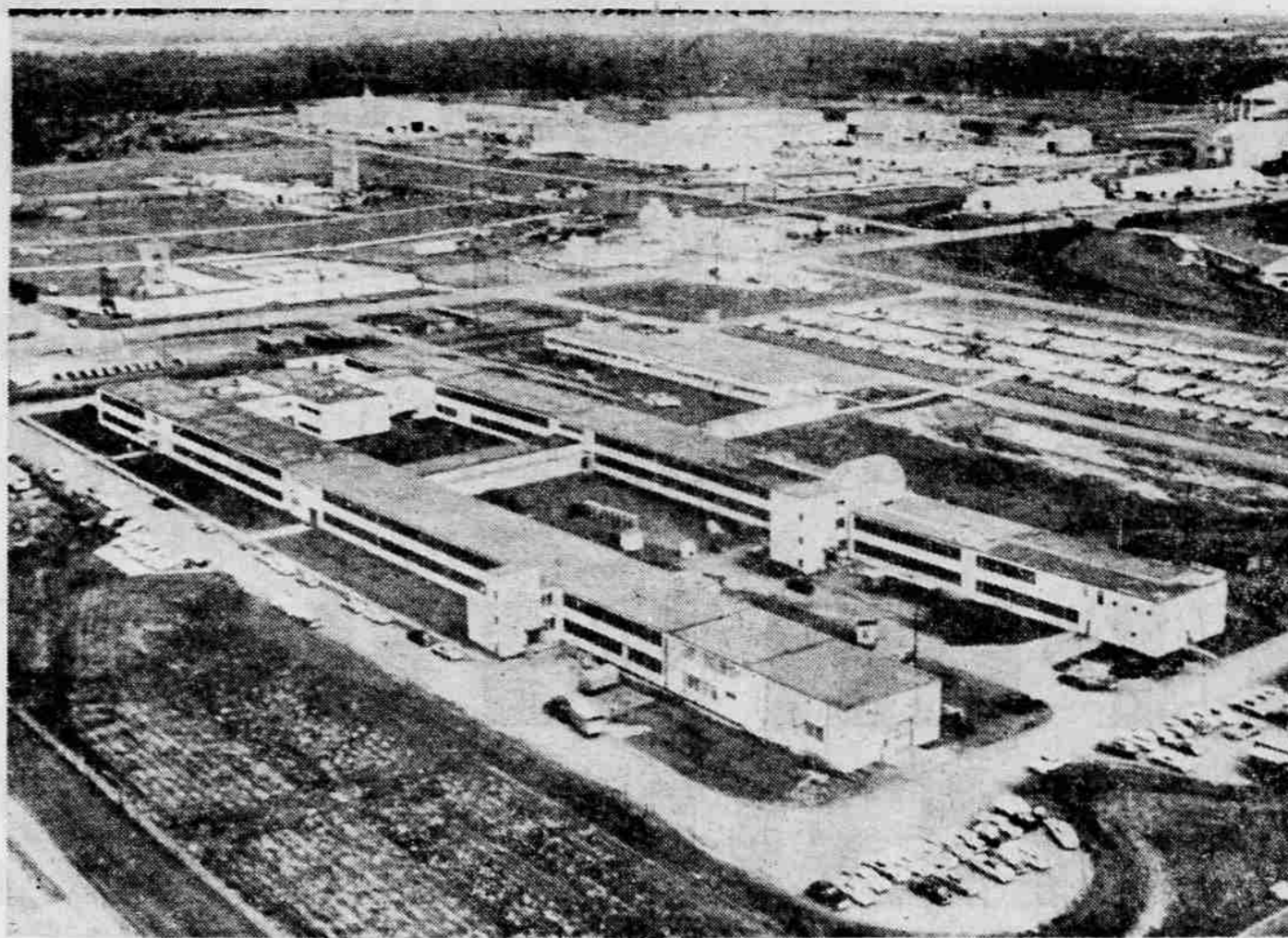
TO TRANSFER FACILITIES—This is an aerial view of a portion of the facilities at Huntsville, Ala., which are to be transferred to the National Aeronautics and Space Administration July 1 under terms of a Presidential proposal announced last October. It will be known as the George C. Marshall Space Flight Center. The facilities, occupied by 10 laboratories headed by Dr. Werner von Braun, are valued at about $100 million. (UPI Telephoto)
