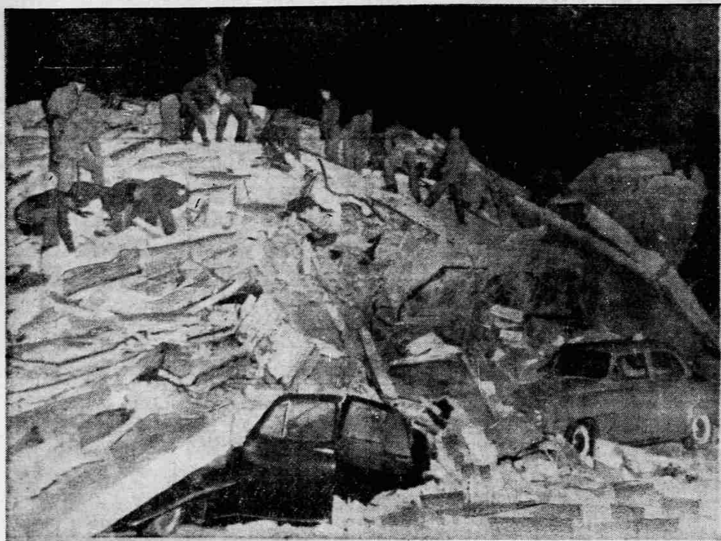
RUBBLE PROBED —U. S. servicemen probe the rubble of a toppled 10-story apartment building in the Talborg area of Agadir, Morocco, where some 300 persons were believed killed by earthquakes that ravaged the city this
