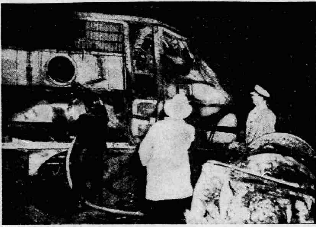
ENGINE DAMAGED — This is the engine exploded, derailing and setting fire to the Santa Fe passenger train that struck an oil truck on a grade crossing near Bakersfield, Calif., Tuesday night. The truck
