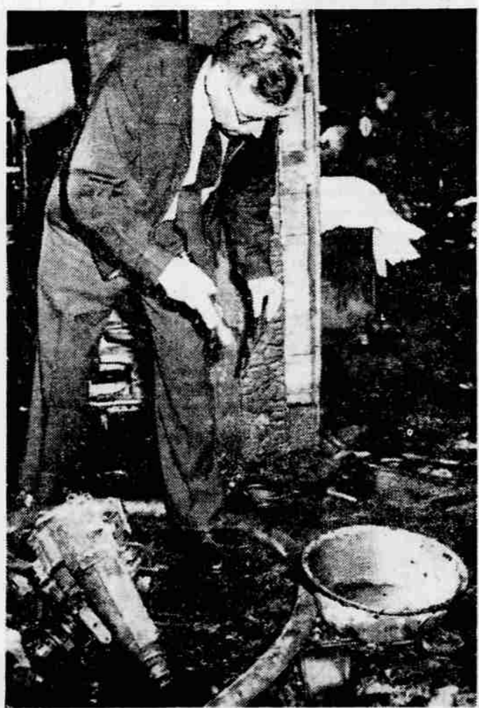
EXPLOSION-FIRE FATAL — Six persons were killed and four were injured in an explosion-fire in a Wichita, Kan., residence, caused when one of the residents was cleaning automotive parts in gasoline. A Wichita fire inspector is shown inspecting a dishpan which contained the gasoline. One of the car parts is shown at lower left.—(UPI Telephoto)
