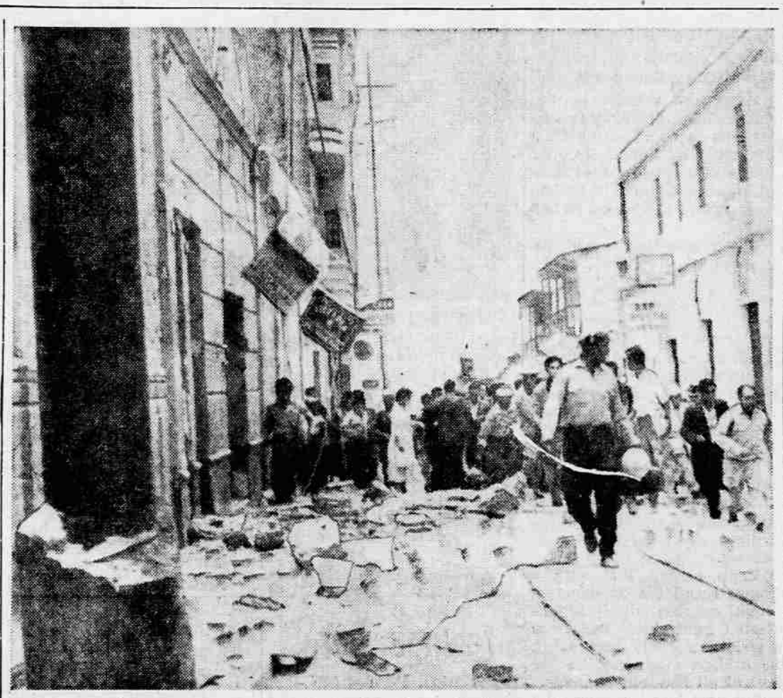
EARTHQUAKE DAMAGE —A shattering earthquake—the worst disaster in the history of Arequipa, Peru, killed at least 38 persons Wednesday and injured more than 200. This is a street scene in Arequipa, showing rubble and wrecked shops. Story on page 2.
