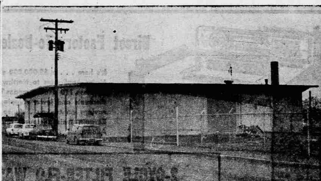
NEW WAREHOUSE - Above is the new warehouse of the Medford school district, which was constructed recently on Columbus ave. The building is part of a two-year construction program approved by the voters in 1957. It will house the district's bus shop. It is tilt-up wall construction.
