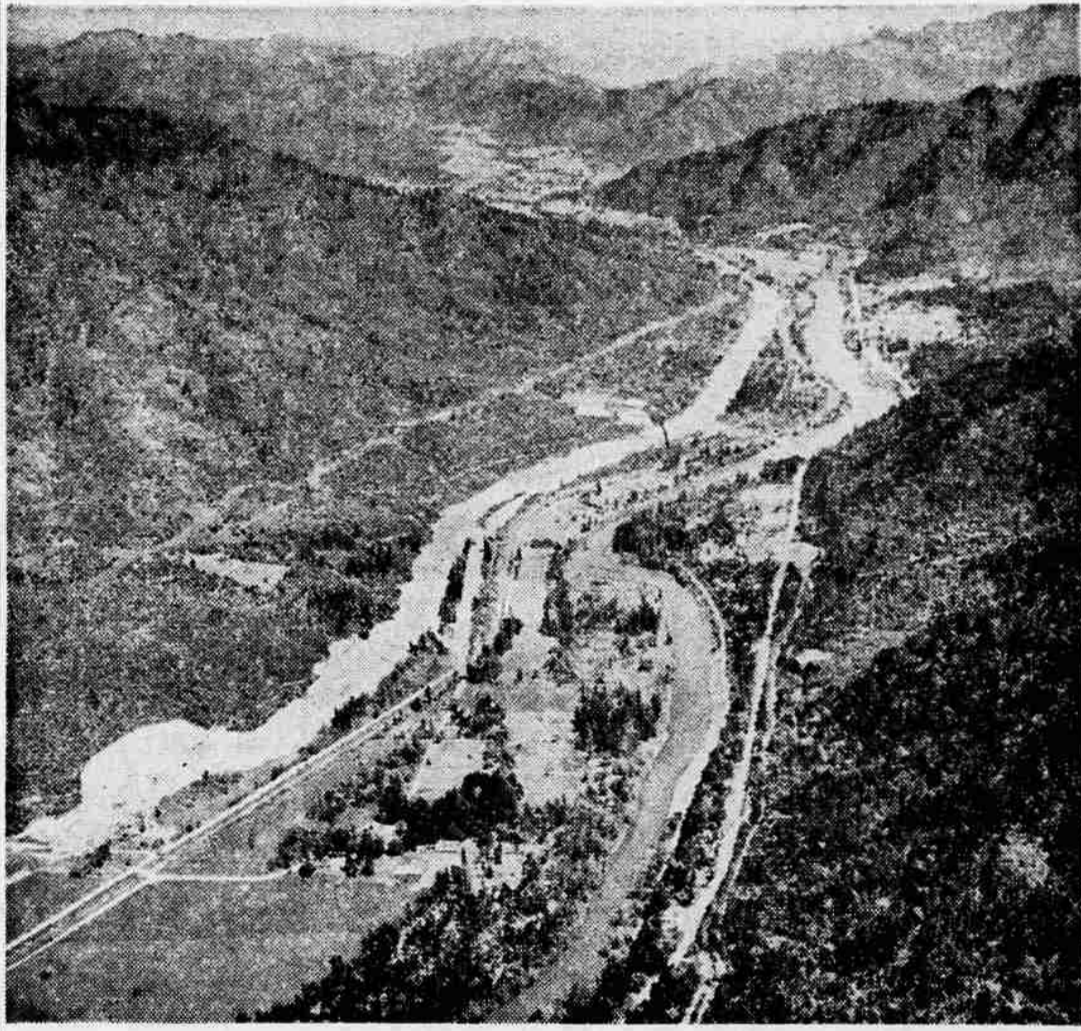
ROGUE RIVER SECTION —Above is a section of the Highway 99 freeway between Grants Pass and Homestead on the Rogue near Gold Hill. An estimated $4,500,000 will be let in contracts on the section this year, the state highway department said. Grading is expected to be completed, and paving and structure contracts are expected to be let. The project was one of several major projects on state highways in 1959.
