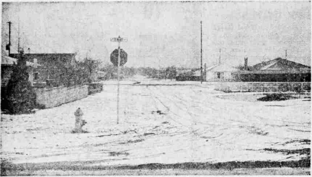
COLUMBUS AVE. —This view of Columbus ave. looking north from Stewart ave. shows the present condition of this street. There is only a light gravel surface here now, but starting in 1961 Columbus will be paved and widened to four lanes from Stewart ave. to McAndrews rd. A section of Columbus has been completed between Jackson st. and McAndrews rd.
