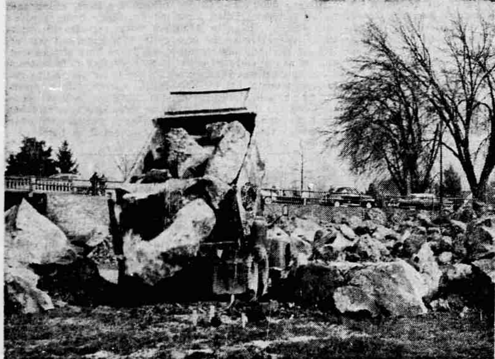
... fill material for new bridge approach ...
