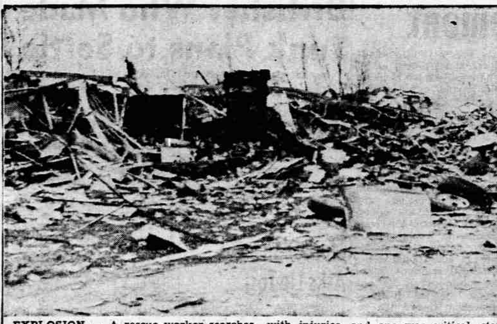
EXPLOSION - A rescue worker searches through wreckage of a bottling plant after it was leveled by an explosion in Warsaw, Ky., Friday. The blast destroyed an estimated 15 homes and damaged 30 others. At least 11 persons were taken to hospitals with injuries, and one was critical, state police said. Eight had been released. The explosion reportedly was caused by propane gas leading from a furnace. (UPI Telephoto)
