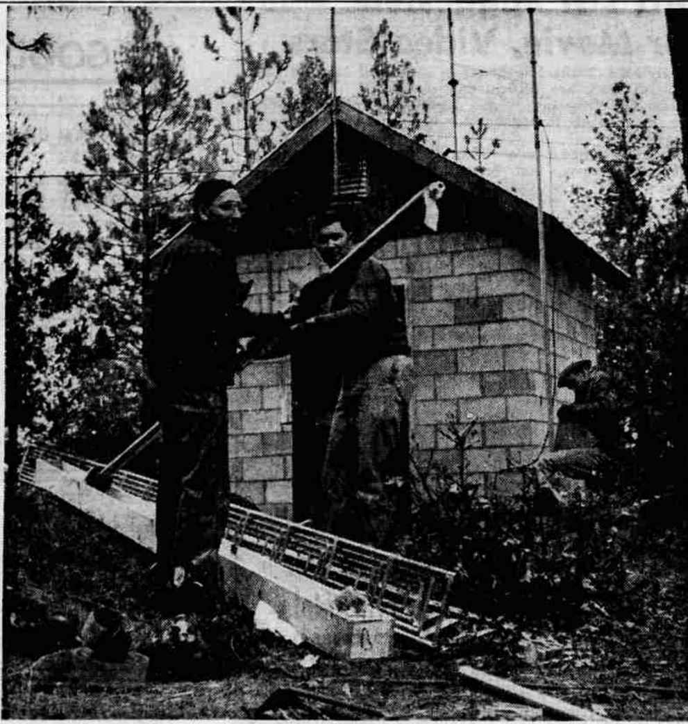
NEW TOWER —A new radio tower, 20 feet taller than the old one, was erected on top of Roxy Ann butte this week to bring greater radiated power to Radio Roxy, southern Oregon's "woods" communications system, and bring increased service to fringe area operators. Above, Dale Prentice, secretary-manager of Southern Oregon Conservation and Tree Farm association (left), and Elk Lumber Company Technician Tom Win-
