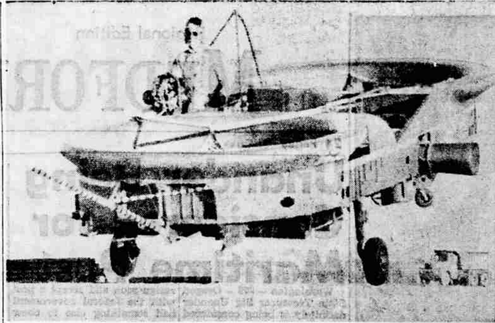
AERIAL JEEP —The world's first aerial jeep is piloted during final tests at Philadelphia by Bob Kennedy of Piaseka Aircraft Corp., which built the jet-powered craft as a prototype for a field test model to be built for the Defense Department. The sky-car combines features of the ground jeep with those of a small helicopter. It is lifted by horizontal rotors at the front and rear. —(UPI Telephoto)
