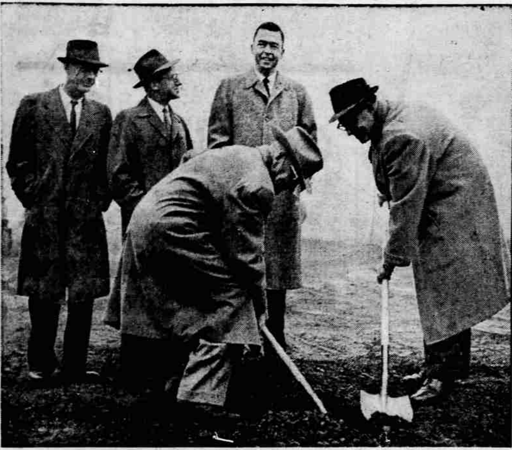
BREAK GROUND—Construction of the new Jackson County Federal Savings and Loan association building in downtown Medford got under way officially this morning as Mayor John Snider, right, and the firm's president, W. J. Warren, turned back shovelfuls of earth. Also pictured above are, left to right, County Judge Earl Miller, Jerry Latham, president of the Jackson County Chamber of Commerce, and Jack Edson, architect for the building. The site is located between Front st. and the railroad tracks south of Main st. Heavy machinery has been doing leveling work there for several days and at one point an old brick walk, a relic of Medford's early days, was unearthed.
