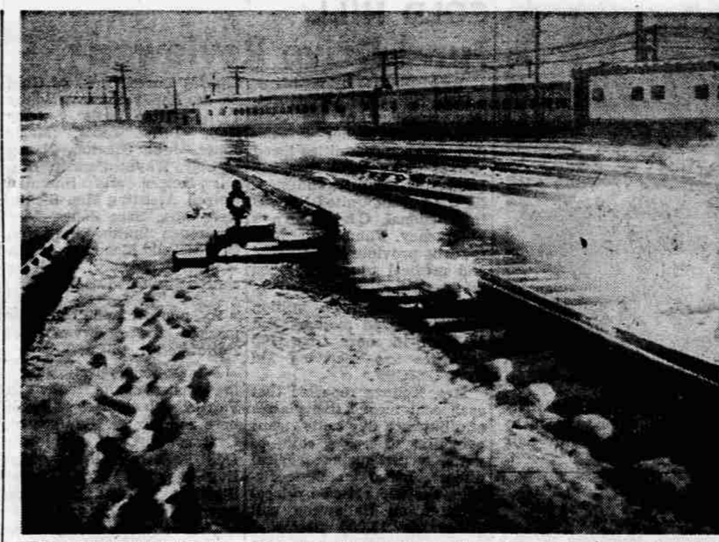
FREEZING PREVENTED —Railroad tracks switches from freezing. Temperatures and ties seem to be ablaze at Chicago as dropped below freezing and four inches flames from burners are used to prevent of snow fall on the area.—(UPI Telephoto)
