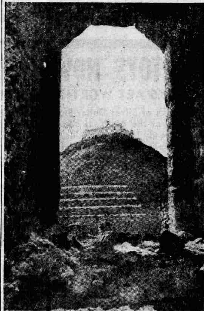
WINDOW FRAMES ABBEY - The abbey of Montecassino standing high on its hill is framed by a shattered window in one of the few walls left standing in the smaller structure below, American fliers plastered the monastery and its basilica with bombs in 1944. Since the war, the Italian government has spent more than $3 million on reconstruction of monastery buildings. (UPI Telephoto)
