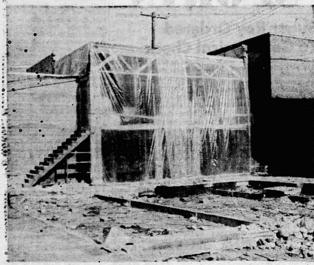
BUILDING SITE —Shown above is the present storage space for newspaper for the Mail Tribune. The new building will be constructed in front of plastic cover, facing Grape st. A 10-foot deep basement will be dug in the area in the center of the picture. The building which was torn down housed Commercial Printing company.
