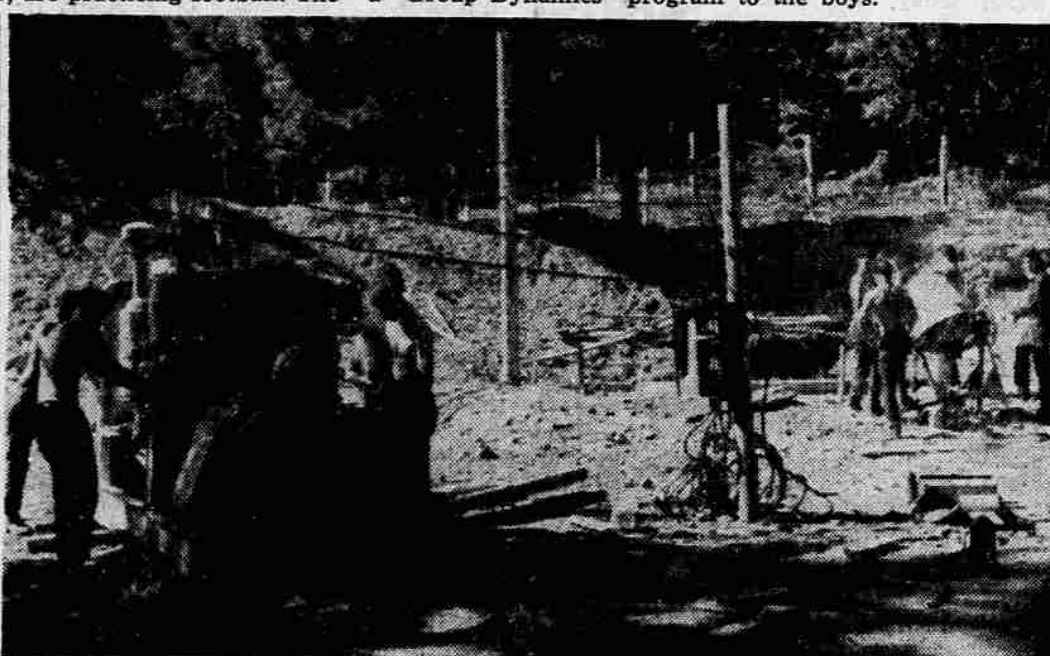
GENERATOR —Boys at the Bar O Ranch are shown getting a new diesel generator in place at the ranch. Those at the right have poured concrete for a base, while others move the diesel generator into location. Boys constructed the site, installed the power poles, and will build the enclosure for the generator. The generator will furnish electricity for the ranch.
