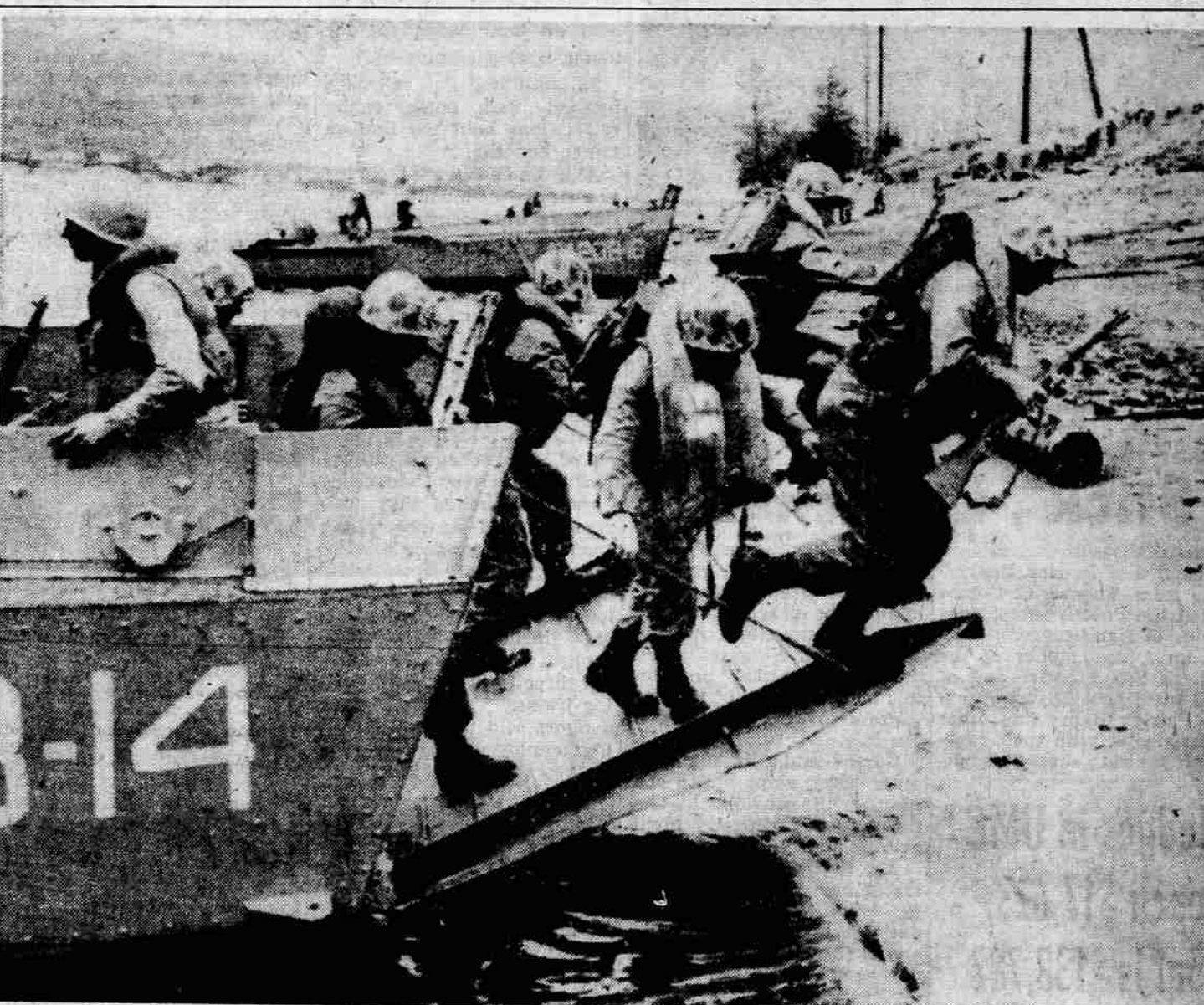
MARINES IN ACTION —Two hundred battle-clad Marines of Portland's 3rd Engineer Reserve Battalion hit the beach and swarmed up nearby Swan Island to establish a beachhead in the first landing and assault operation ever conducted in the Portland area. —(UPI Telephoto)
