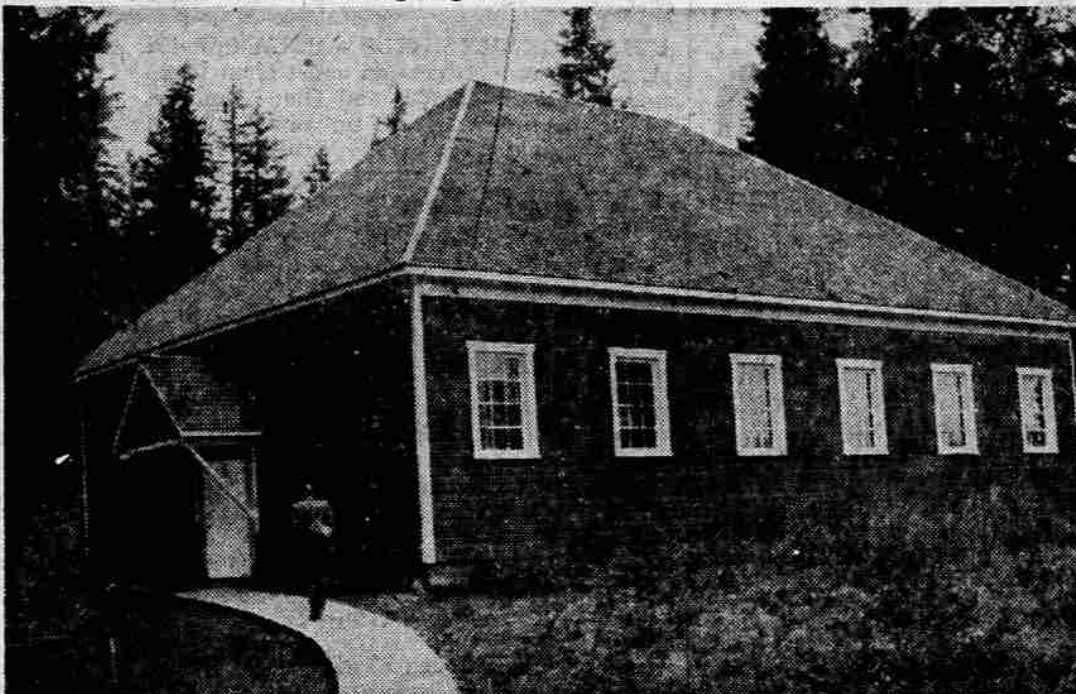
PLAYSHED - Assistant County School Superintendent Bruce Hitt ambles up the cement path to the Pinehurst school playshed. Unheated and with rough floors, the building is not up to standards set for school gymnasiums so must be designated a play-
