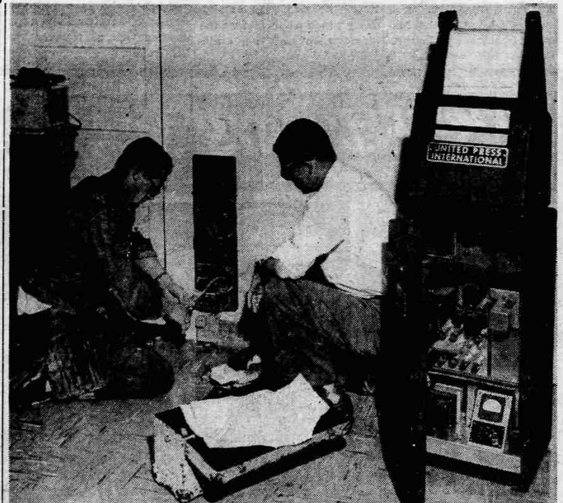
MACHINE INSTALLED — Roy Davenport, right, telephoto engineer from United Press International offices in San Francisco, was on hand to check the operation of the new Unifax receiver installed at the Mail Tribune this morning. Wiring in the machine, left, is H. R. Parrott Jr., an employee of
