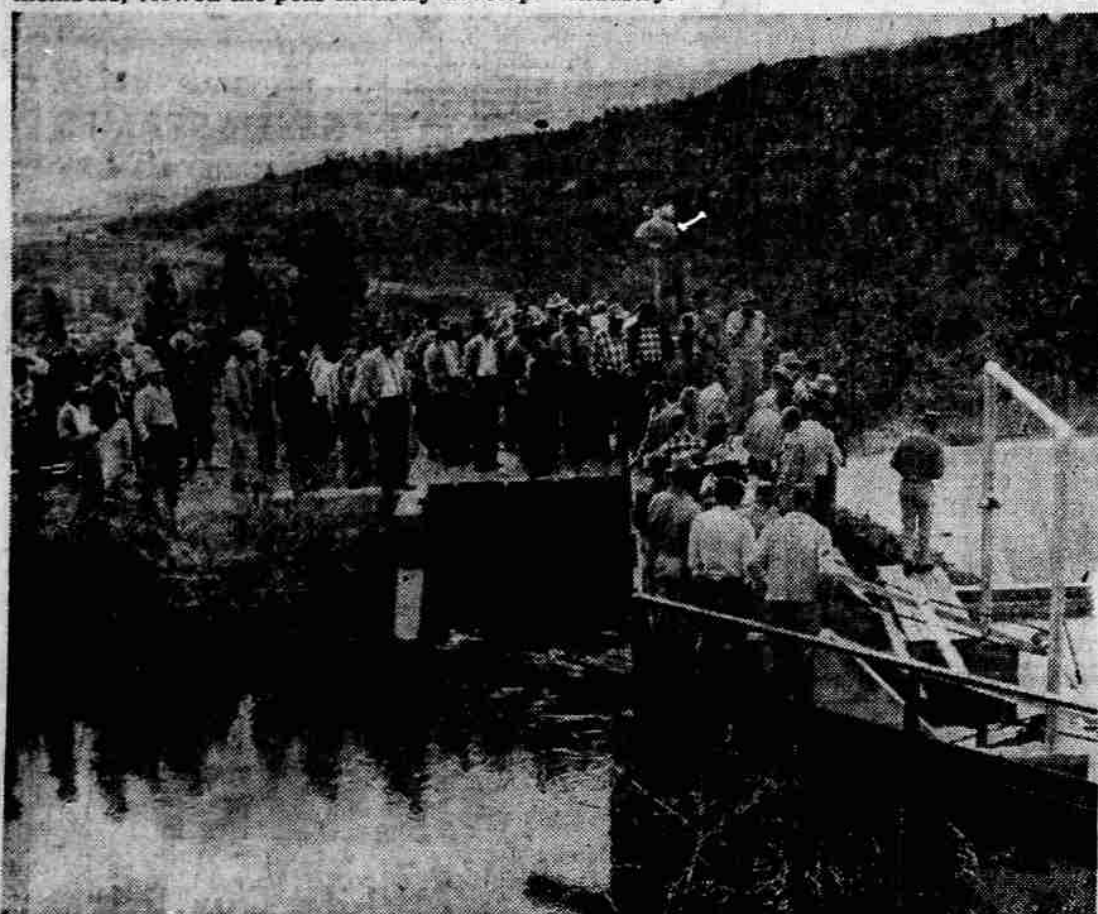
VIEW FOREBAY —Ted Flury, Eagle Point Irrigation district manager, led a tour through the district's power plant forebay near Nichol's gap yesterday afternoon during the annual conference of irrigation oper-
