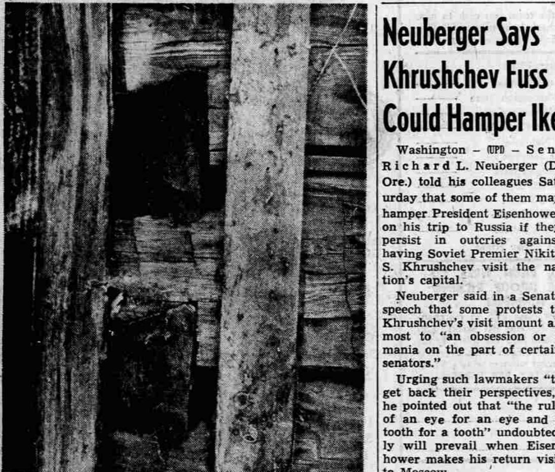
CORNER JOINTS - This unique joint used in the construction of the Ziegler home on the Applegate, built in the 1870's, makes a flush corner, eliminating projecting ends of the logs. Careful fitting was necessary to get the joints to "seat" properly. The logs themselves were hand hewn to create a flat surface inside and out.
