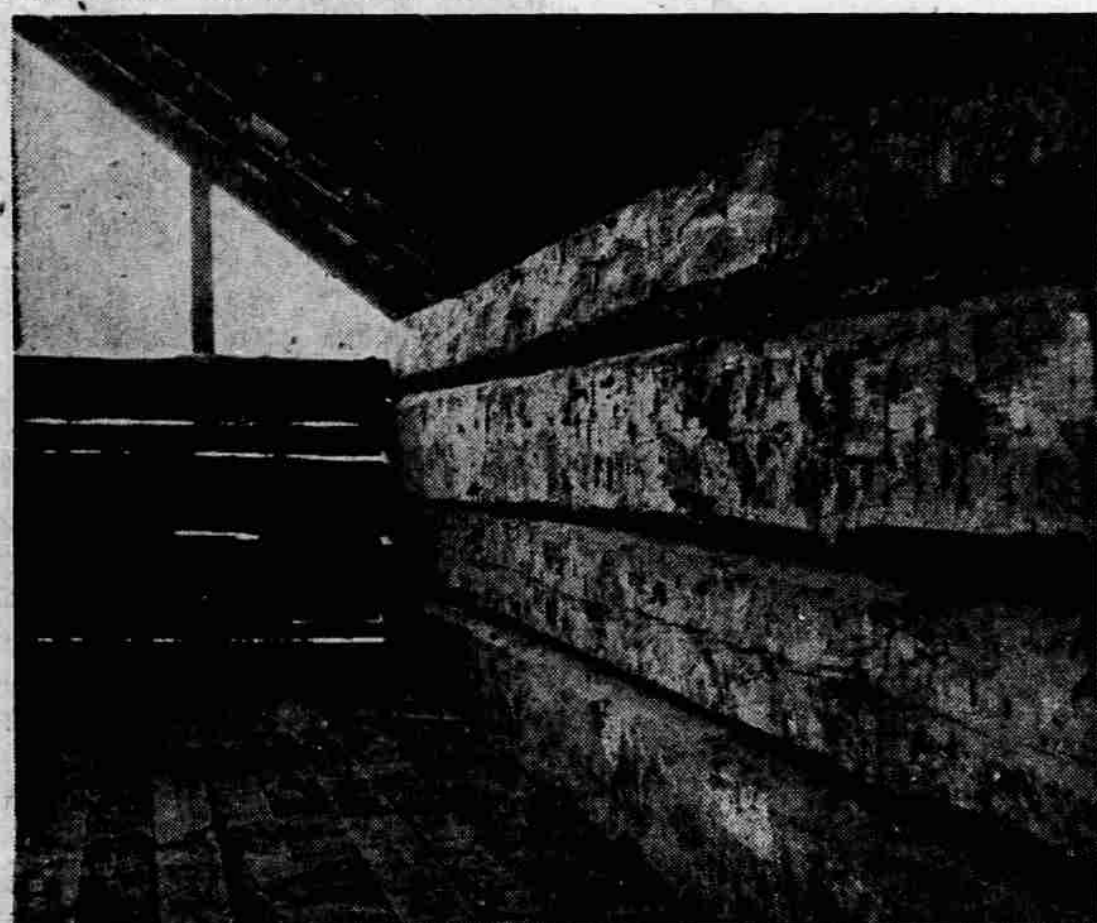
UPPER FLOOR - The upstairs room in the log home owned by Mr. and Mrs. W. H. Ziegler used to be a snug attic bedroom, but has not been used for many years. The logs show clearly the marks of the axe that was used to shape them. Rafters in the building are of poles and "sawed" boards were used as support for the shakes that originally covered the roof. Ziegler recently tore the siding off the building, exposing the open gables above the log construction.
