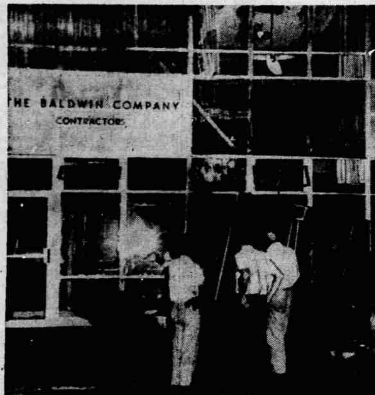
WRECKING TWO OFFICES and fire chief's car, three bombs startled Little Rock, Ark., center of anti-integration turmoil. This is damage to office building containing private offices of mayor. School Board buildings also suffered extensive damage. No one was injured.
