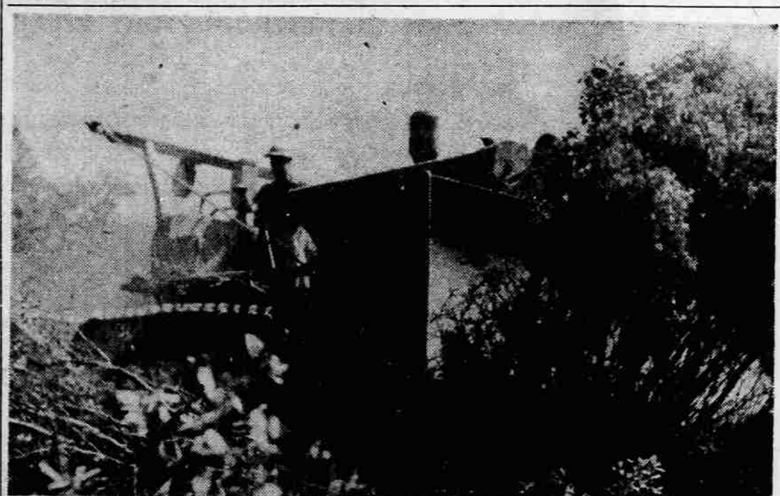
PUSHES THROUGH - The giant D-8 Caterpillar tractor pushes down some brush with its giant blade on O and C land in the Applegate area. A giant root-plow attached to back slices through the brush roots. Much of the time the tractor operated on a 50 per cent grade - a grade few cars can pull up.
