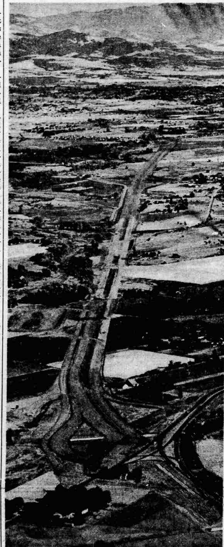
FREWAY CONSTRUCTION -This is a view of the Highway 99 freeway construction from just south of Central Point (upper part of photo) to the intersection with the present Highway 99 and old 99 south of the Tolo overpass. The interchange construction toward the top end of construction area is the Central Point interchange. The picture was taken by Kenn Knackstedt, Medford photographer.
