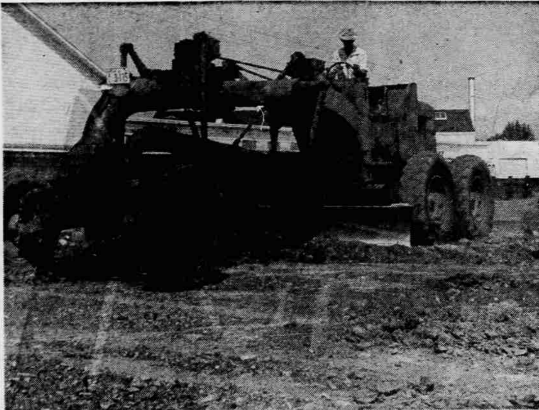
GRADE SCHOOL GROUND —Art Stinson, grader operator for Contractor Ted Florey, grades the Howard school ground in preparation for opening of school next month. Material used for fill dirt was that left over when sewer ditches were dug in the Berrydale district. The work was being done in preparation of blacktop paving.
