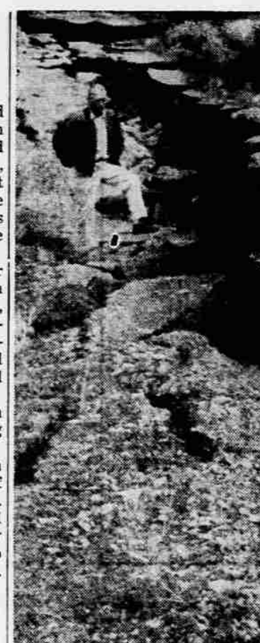
KEEPING QUAKE AREA isolated, gaping cracks in road near Hebgan Lake, Mont., are left by disastrous earthquake that took undetermined toll of human life.
