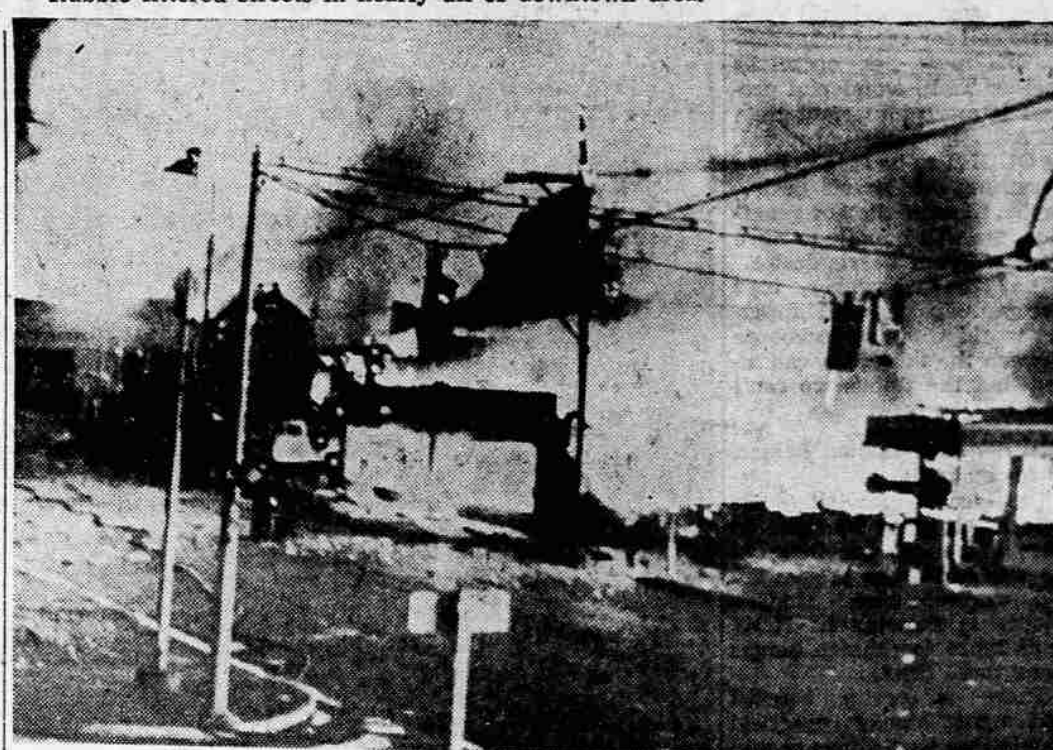
HUGE OREGON EXPLOSION —A truck containing six tons of dynamite and ammonium nitrate blew up in a Roseburg, Ore., lumber yard as a result of a fire. An area of four square blocks was leveled and damage extended for about 20 blocks.
