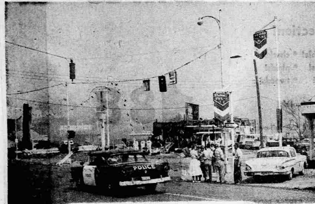
Sober-faced residents discussed the utter destruction.
