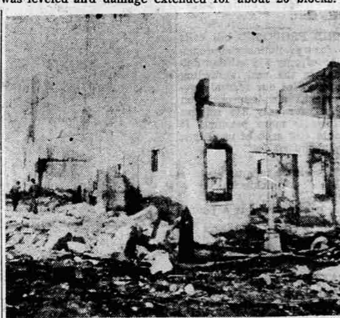
AFTERMATH —A major part of Roseburg, Ore., looked like a bombed out city. Only the shell of this building, two blocks from the center of the ammonium nitrate and dynamite explosion, was left standing.
