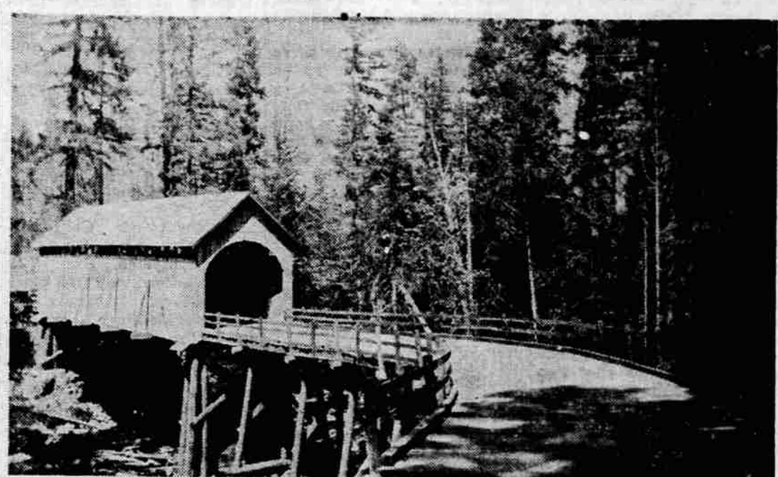
COVERED BRIDGE —This old covered bridge, which still is in use today, was built by the Hartman brothers in 1922. It spans Big Butte creek about three miles below Butte Falls. It is known as the Hawk bridge, after a man by the name of Hawk who asked the county to put it in. Timbers in the bridge are 80 feet long, hand hewn from logs cut on the site.
