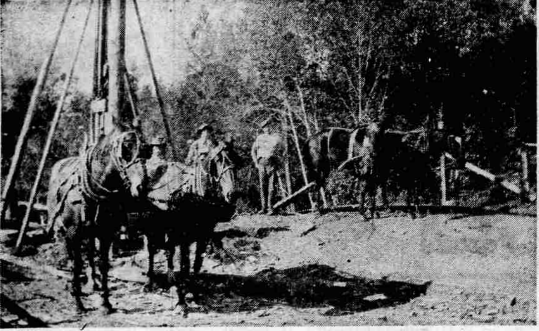
HORSE POWER —In the early days of bridge construction in Jackson county, pilings were driven into the ground by means of a horse-operated "hammer," like the one pictured above. The men are Bill Owings and Bill Moore, who, with their horses, were hired by the day by the county to operate the pile driver. The picture was taken in 1922.
