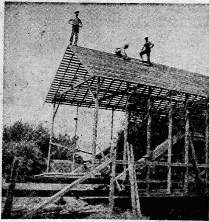
FRAMEWORK —The men above are working on the roof of the Antelope creek bridge, which was built by the county in 1922. Covers over the bridges added little to their strength, but protected timbers from exposure to weather and made them last years longer.
