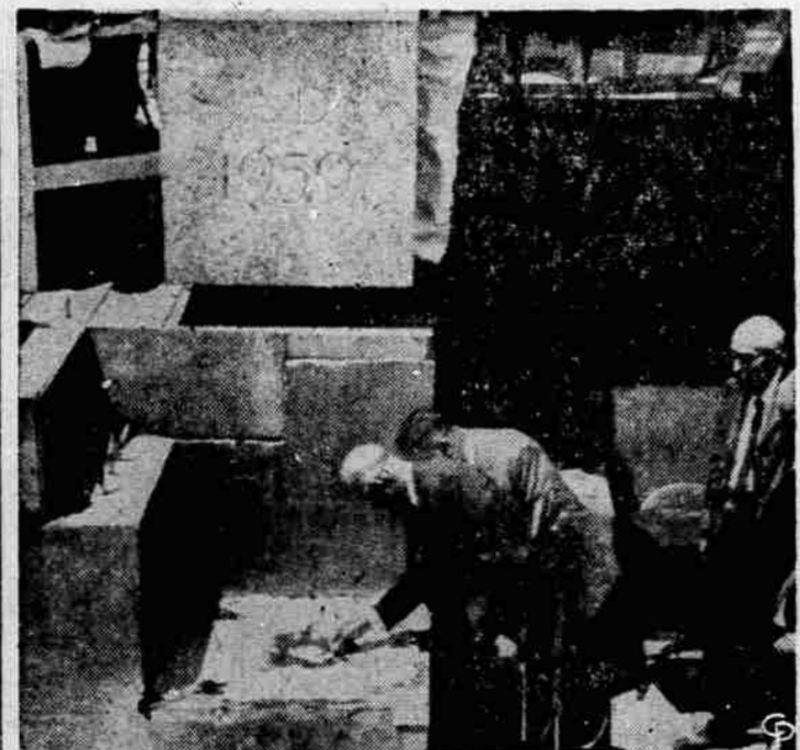
USING TROWEL wielded by George Washington when first cornerstone of Capitol was laid in 1793, President Eisenhower spreads mortar for new cornerstone at East front of Capitol, now being extensively remodeled.
