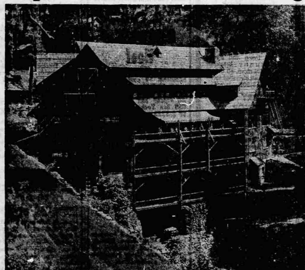
This rustic chateau, nestled against the mountainside, was constructed in 1934 at the Oregon Caves National Monument. Other facilities for overnight guests include a three-story chalet and seven cottages. No camping is permitted in the national monument area.
