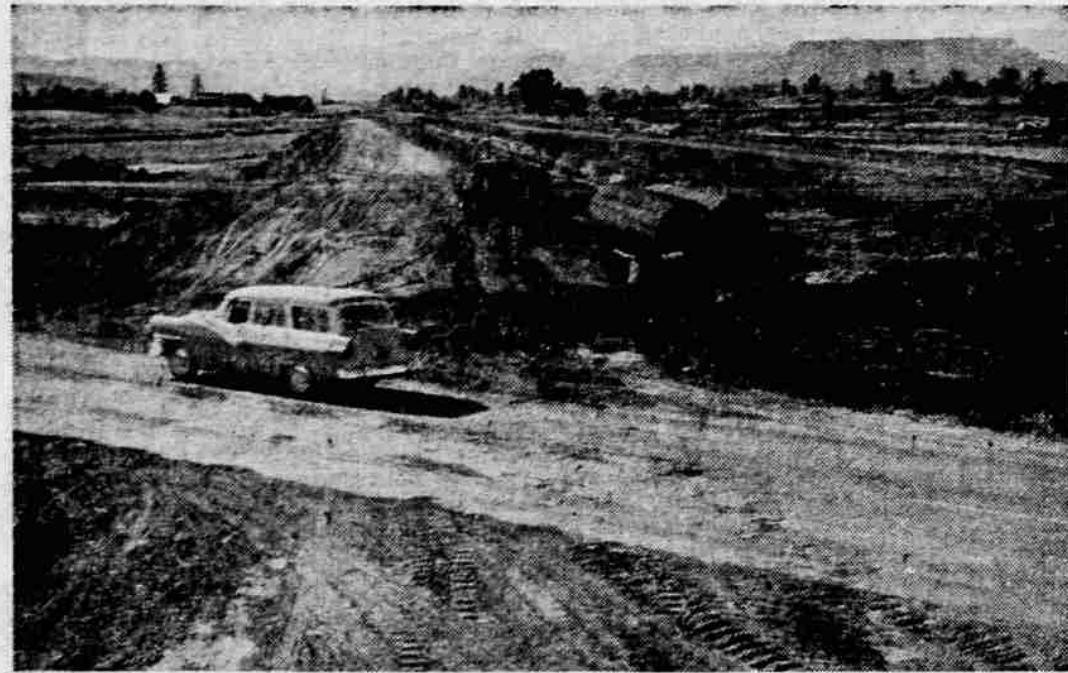
Freeway construction in Central Point area ...
