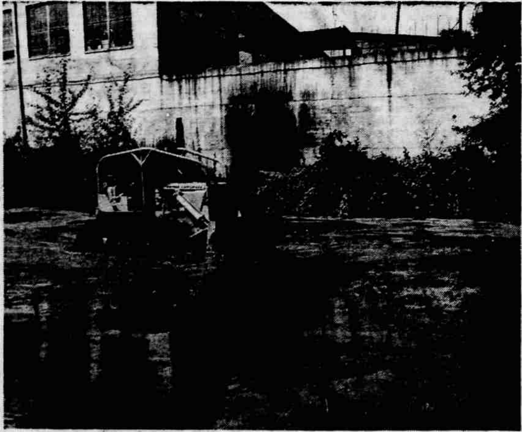
SPRING CLEANING —The Bear creek channel received its annual cleaning Wednesday morning when the city hired a bulldozer to clean out weeds and debris between the Cottage st. and Jackson st. bridges. City Manager Robert A. Duff said that the clean-
