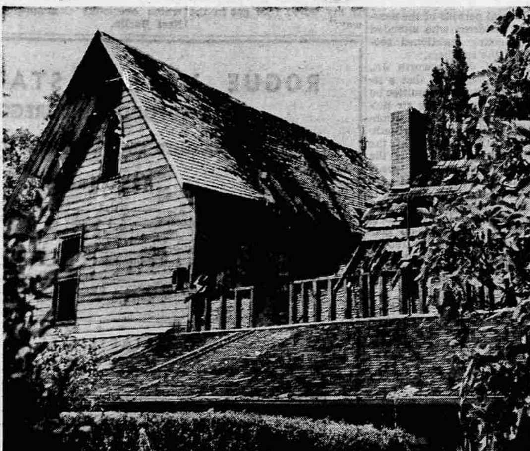
BRITT HOME - The fire April 29, 1957, gutted part of the house built by Peter Britt, pioneer photographer, nearly 100 years ago has made the property more than a "white elephant" for its present owner, Southern Oregon college. Britt's former studio on the left now has two skylights, one of glass and the other of charred wood.
