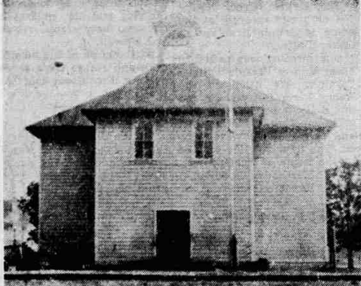
EAGLE POINT SCHOOL - The first floor of the Eagle Point school building shown above still stands. It was constructed in 1900. The history of the Eagle Point consolidated district starts at the same time the Jacksonville district was organized, in 1854.
