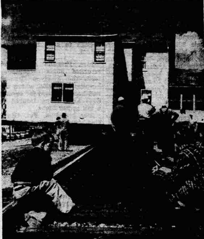
RAILROAD —The railroad doesn't really run through the middle of this house in LaCrosse, Wisc. The building is being moved across the tracks, and the movers were able to get it moved before any traffic came along.
