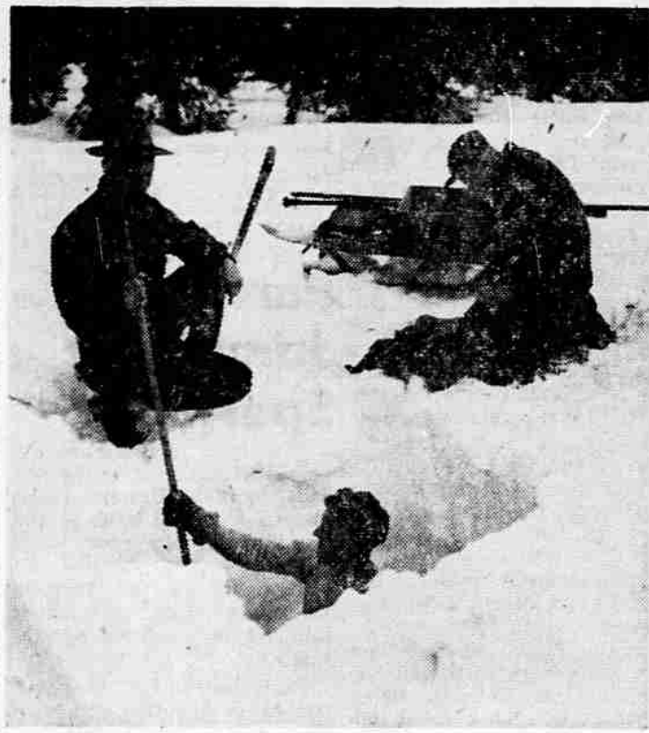
SOIL SAMPLE —Early efforts by Oregon cooperative snow surveys to improve accuracy of seasonal water supply forecasts included physical collection of soil samples from earth beneath snowpack. The samples were weighed, oven-dried and reweighed, and the moisture percentages computed. This picture was taken about 1938 in Crater Lake National park. Left to right are R. A. Work, R. W. Childreth and G. F. Sturdevant.
