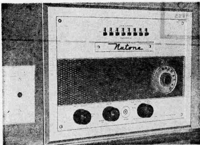
Sound-control center is located in the kitchen . . . with speakers in all three bedrooms and on the veranda. You can speak from the kitchen to any of these rooms . . . or any of the rooms can contact another room through the speaker system. It also allows a busy mother to listen to any of the rooms . . . or outdoors . . . to be sure the children are safe. The outdoor speaker acts as a watchman at night. The system is already set to transmit AM and FM radio to all rooms (which have independent volume controls) . . . and has a plug-in for phonograph connection. Handy plug-in for portable telephone is located next to the sound-control center.
