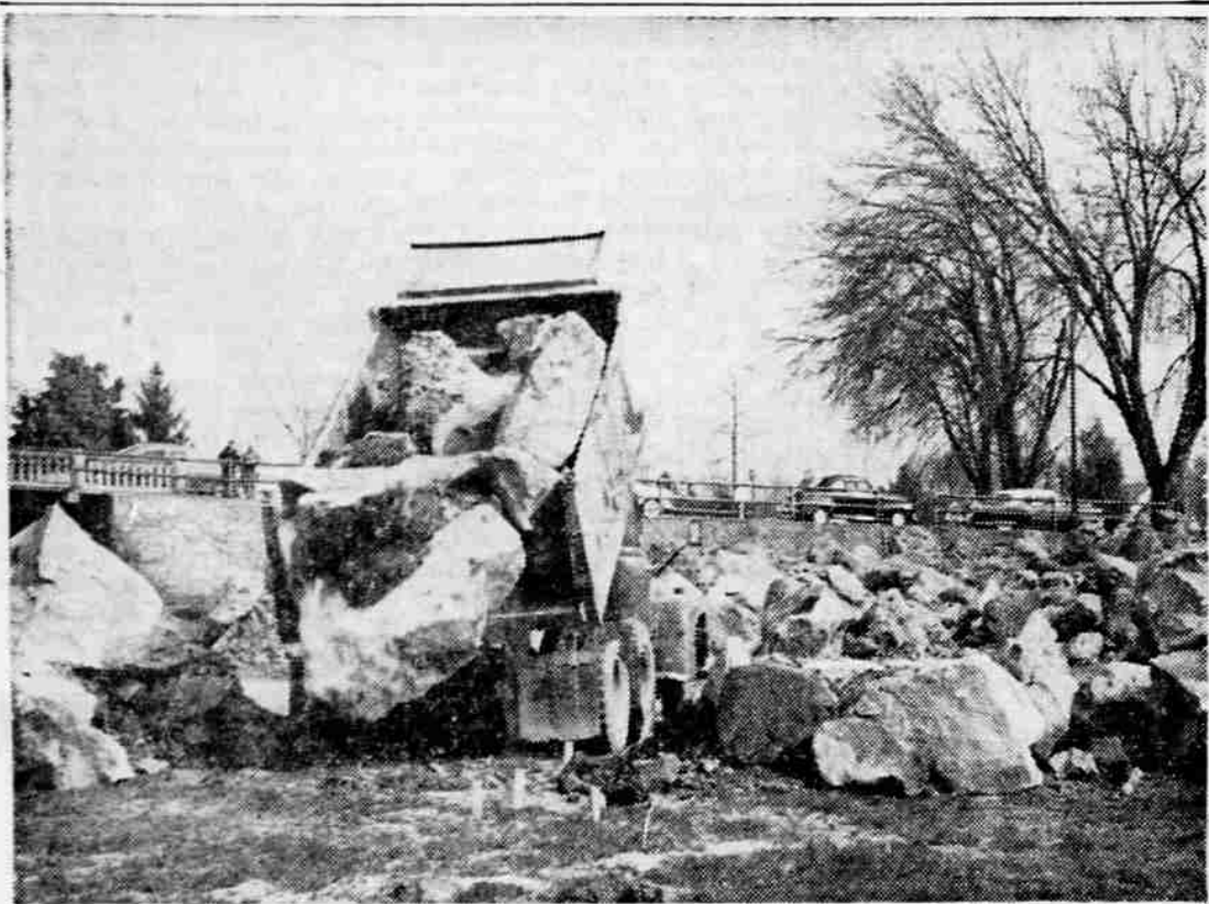
FILL ROCK —Above, a truck dumps its load of huge boulders, removed from the Rogue Valley manor site on Barneburg hill, which will form the base support for the Eighth st. extension fill near the Scout office on East Main st. A reinforced concrete bridge will span Bear creek from where the fill ends. Sidewalks will be built along both sides of
