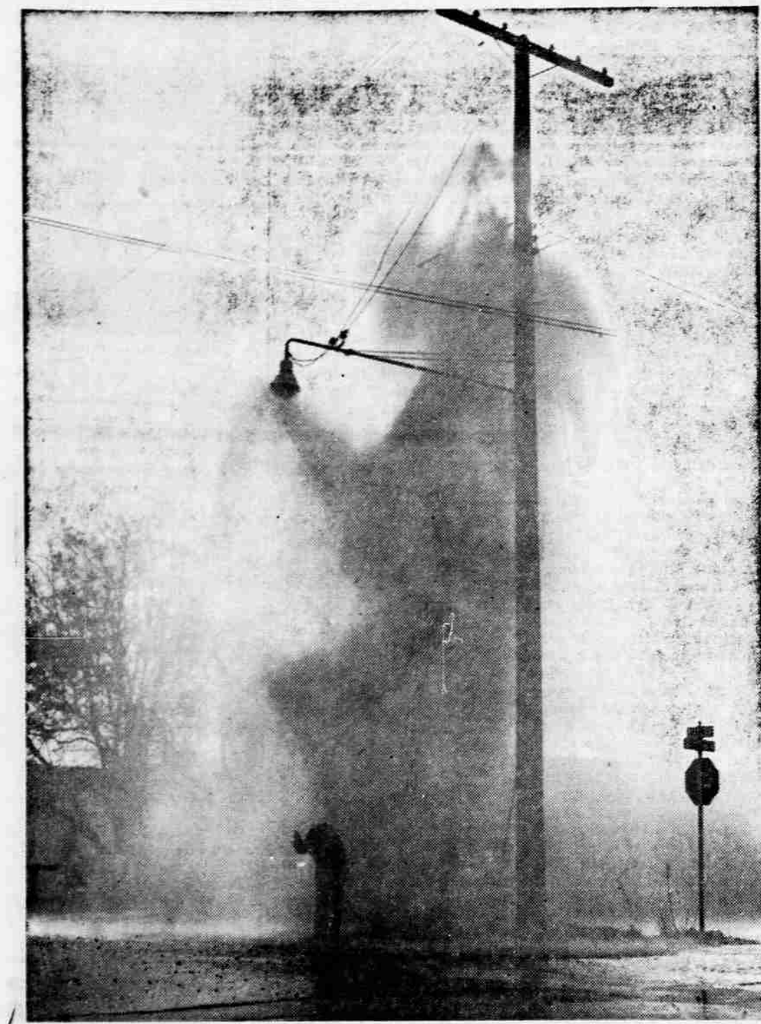
BROKEN MAIN—A 50-foot geyser of water burst from a broken fire hydrant on West Main st. at Jeanette st. at 9:20 a.m. today and spewed water and gravel for 20 minutes before the main serving it was shut down. Medford Water Superintendent Robert L. Lee said the hydrant was sheared off by a California Oregon Power company service truck maneuvering for some drill-
