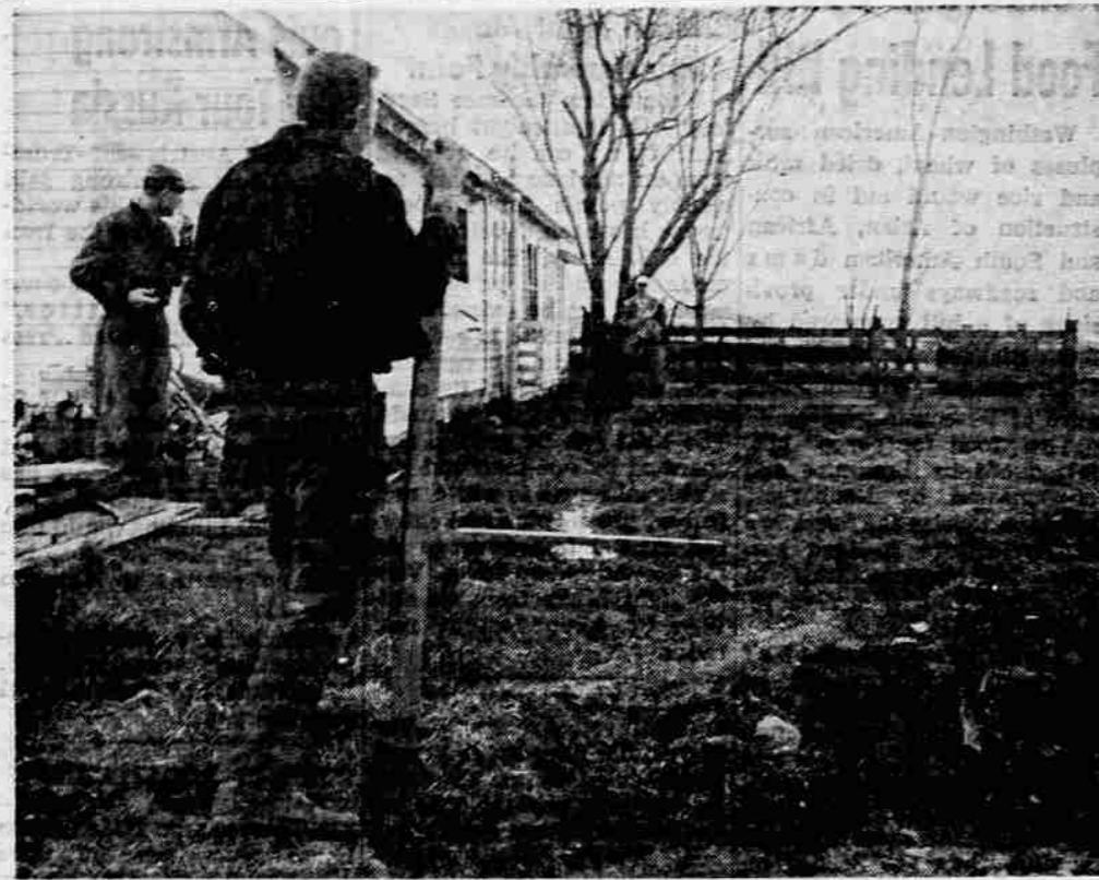
DETERMINE GRADE - Darrell L. Fariss, of the Sanitation Service, assists Jackson County Sanitarian Orié Moore, far right, in getting a rough estimate of the grade near Bud Hoover's house in the Camp White area. Looking on, at left, is Bud Hoover. Strictly on an experimental basis, the Sanitation Service will connect a septic tank with an evaporation type of drainage field at the Hoover home. Effluent from the septic tank will be carried through pipes to gravel spread 18 inches deep on top of the ground and will be allowed to evaporate. Usual method is to carry the effluent to drainage fields below the ground surface.
