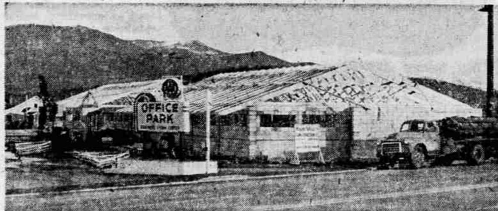
BLM OFFICES—This new building, going up at 1133 South Riverside ave., Medford, will house the office of the bureau of land management. It has been located in the city hall for more than 20 years. The new building, measuring 44 by 206 feet, will contain 14 offices joined by a hallway leading both directions from the main entrance. The structure is being built with shale brick and will feature glass brick "windows." It is in Office Park, South Riverside ave. and Barnett rd., owned by O. L. Williams, who is building it to General Services administration specification. The BLM is scheduled to occupy the new building before April 1, according to District Manager Ross Youngblood.
