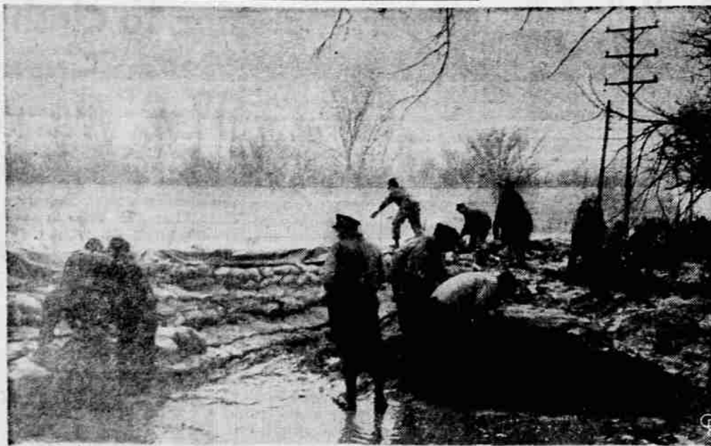
SANDBAGGING THE WABASH RIVER , these Indiana National Guardsmen, Air Guardsmen and inmates of penal institutions are trying to control the rising flood waters near Terre Haute. A round-the-clock effort is being made to prevent flooding of city, partially evacuated as a precautionary measure. Dike is over four feet high, six feet thick, and was resisting surging floods. River rampage aided by storms.
